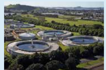
The Mangere Wastewater Treatment Plant treats about 75% of Auckland's wastewater.
