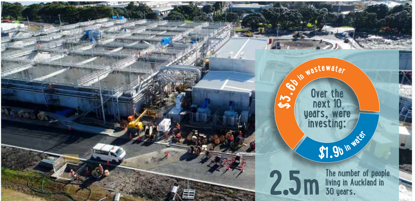
An aerial shot during construction of the biological nutrient removal facility at the Māngere Wastewater Treatment Plant, late 2017. Beginning operation in the next few months, this upgrade will enable the plant to cater for Auckland's increased wastewater demand.
