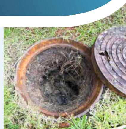
A manhole in a front yard blocked by wipes, rags and fat, caught up on tree roots.
